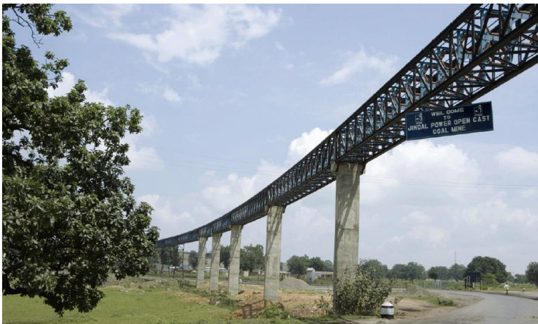
6.9 km cross country pipe conveyor belt for coal transportation
