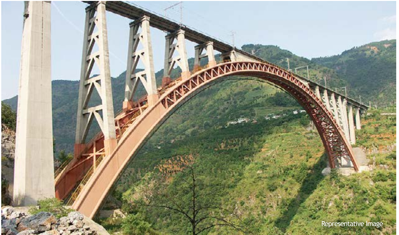
World's Highest Bridge (359M above MSL) with incremental curvature
