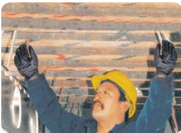
3 Lock bars placed approximately 300 mm apart to give plywood support
