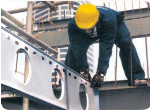
1 Speedfloor joist lifted into place
