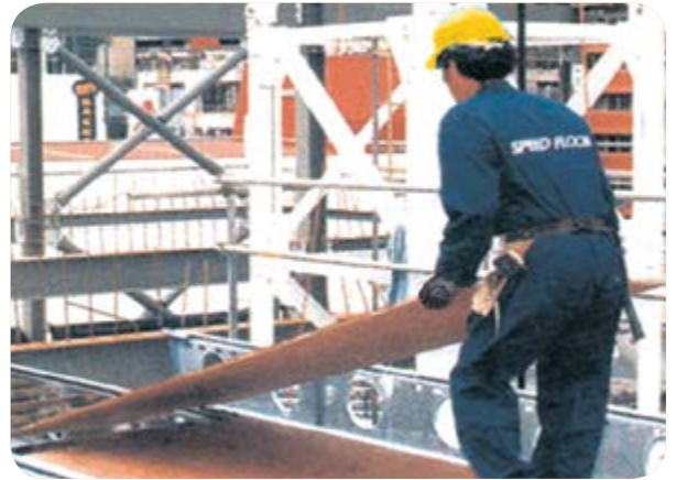
4 Plywood introduced from top
