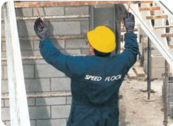
2 Lock bars slide into pre-punched holes to support the plywood shuttering
